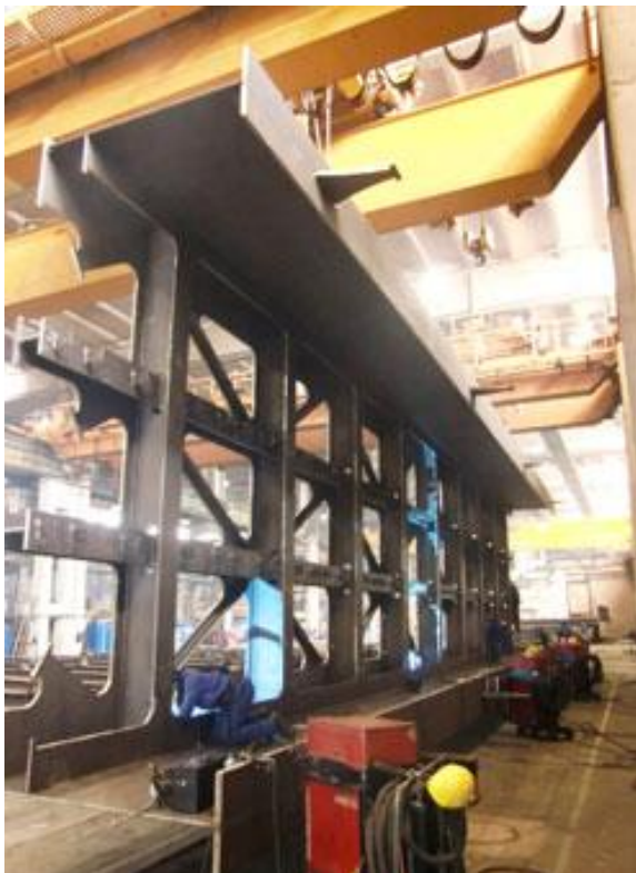
Figure 2: Large structural steelwork for the 'Hafenbahn Magdeburg/Germany'
