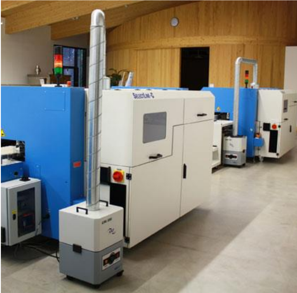
Image 3: LRA 200 fume extraction unit with flexible piping to SEHO soldering systems
